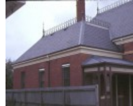
numurkah court house melville street numurkah side elevation nov1984
