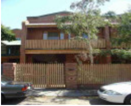
carlton north henry street carlton north henry street 9
