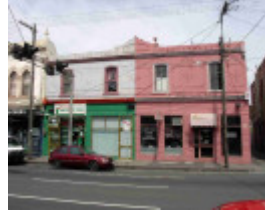
Collingwood Johnston Street 85-91.JPG
