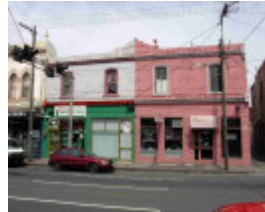
Collingwood Johnston Street 85-91.JPG
