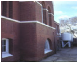
former omeo post office side wall jul1980
