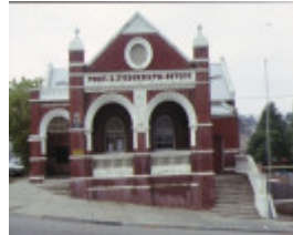
former omeo post office front view
