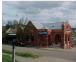
former omeo post office corner view oct1999
