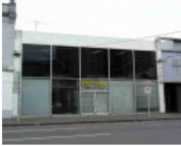
collingwood johnston street collingwood johnston street 192-194
