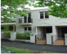
richmond elm grove richmond elm grove 27 unit 1
