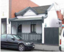
collingwood emma street collingwood emma street 21
