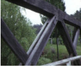
hinnomunjie bridge omeo detail of wooden beams
