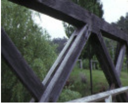
hinnomunjie bridge omeo detail of wooden beams
