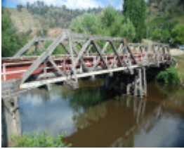
HINNOMUNJIE BRIDGE SOHE 2008
