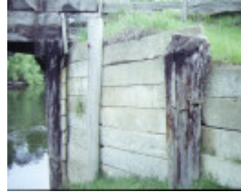
hinnomunjie bridge omeo river bank supports
