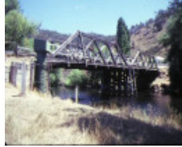
1 hinnomunjie bridge omeo side view feb1985
