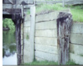
hinnomunjie bridge omeo river bank supports
