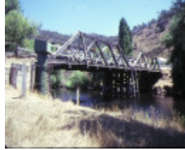
1 hinnomunjie bridge omeo side view feb1985
