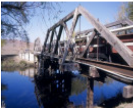
h00917 hinnomunjie bridge over mitta mitta river omeo steel upright installed she project 2003
