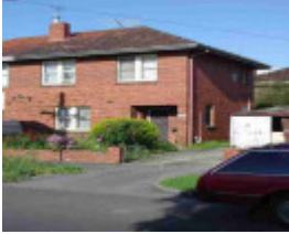
burnley tudor street burnley tudor street 41
