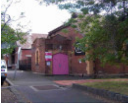
Richmond Church Street 314C.JPG
