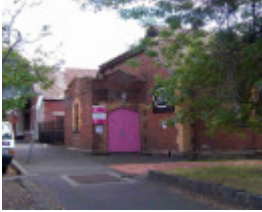
Richmond Church Street 314C.JPG
