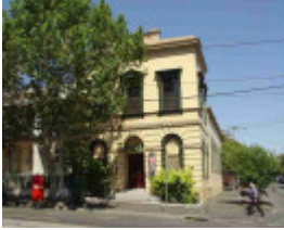
richmond church street richmond church street 316
