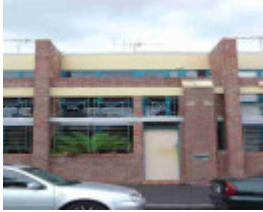
princes hill holtom street princes hill holtom street 8
