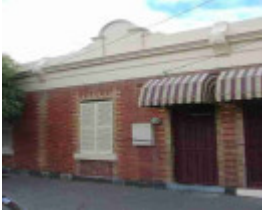
carlton north park street carlton north park street 312
