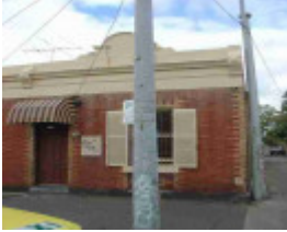
carlton north park street carlton north park street 316
