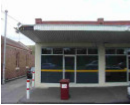
carlton north park street carlton north park street 320
