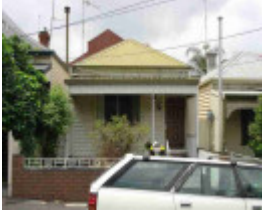
cremorne cubitt street cremorne cubitt street 183
