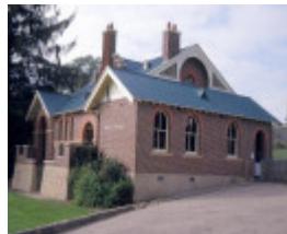
h01536 omeo justice precinct day avenue omeo 1893 courthouse western side
