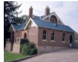
h01536 omeo justice precinct day avenue omeo 1893 courthouse western side
