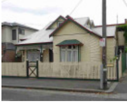
princes hill holtom street princes hill holtom street 17
