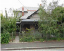
princes hill holtom street princes hill holtom street 29
