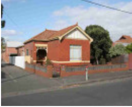
princes hill holtom street princes hill holtom street 75
