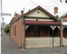
princes hill holtom street princes hill holtom street 81
