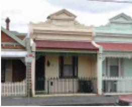
princes hill holtom street princes hill holtom street 85
