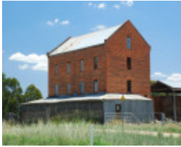
FORMER FLOUR MILL SOHE 2008
