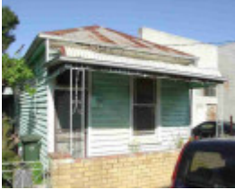
collingwood dight street collingwood dight street 22
