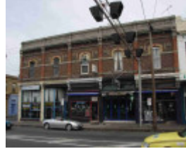
Collingwood Johnston Street 5-11.JPG
