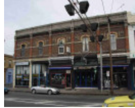
Collingwood Johnston Street 5-11.JPG
