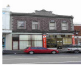
Collingwood Johnston Street 34-36.JPG
