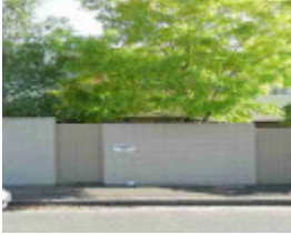
richmond james street richmond james street 25
