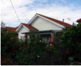
richmond johnson street richmond johnson street 29
