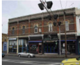
Collingwood Johnston Street 5-11.JPG
