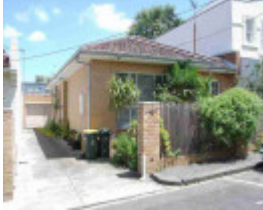
richmond rogers street richmond rogers street 2
