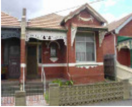
carlton north station street carlton north station street 580
