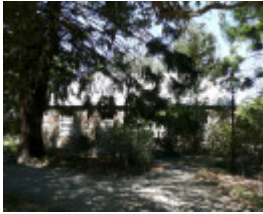
FORMER TRAVELLERS REST INN SOHE 2008
