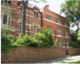
JCH 1891 Main Wing (left) and adjoining 1956 Joske Wing (right)
