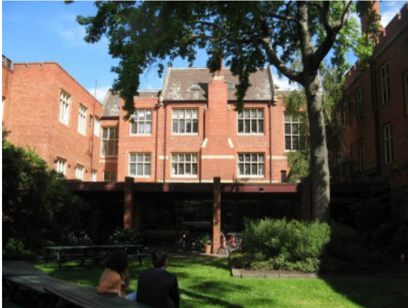
JCH rear (east side) of main wing and courtyard addition
