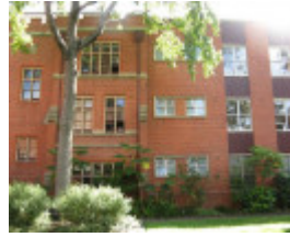
JCH Part of the 1930 Traill Wing (left) and the adjoining 1962 Scantlebury Wing, which form the north side of the courtyard.
