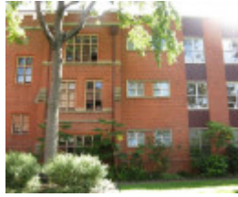
JCH Part of the 1930 Traill Wing (left) and the adjoining 1962 Scantlebury Wing, which form the north side of the courtyard.
