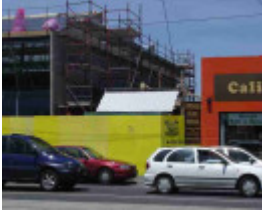
burnley bridge road burnley bridge road 514
