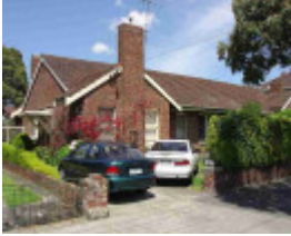
burnley bridge road burnley bridge road 624
