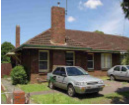
burnley bridge road burnley bridge road 628
