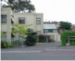
richmond freeman street richmond freeman street 2a
