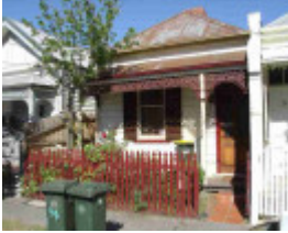
richmond gardner street richmond gardner street 34
