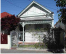
richmond gardner street richmond gardner street 36
