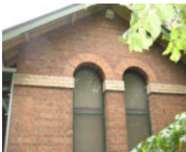
segmental arched window pair to facade
