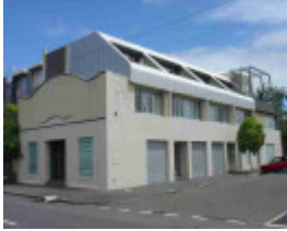
carlton north curtain street carlton north curtain street 1
