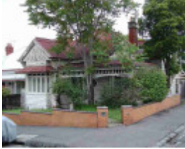
richmond malleson street richmond malleson street 2
