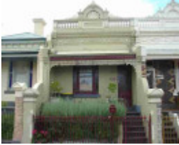
carlton north station street carlton north station street 544
