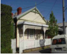
collingwood palmer street collingwood palmer street 58- 60
