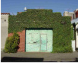
collingwood palmer street collingwood palmer street 62
