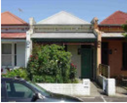
burnley park grove burnley park grove 16
