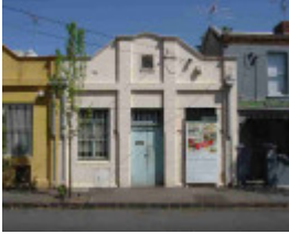
collingwood harmsworth street collingwood harmsworth street 65-67
