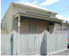
richmond loughnan street richmond loughnan street 6
