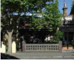
richmond church street richmond church street 249
